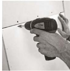
**8** Screw on the speaker according to the pre-drilled holes. The heads of the drywall screws should immerse about 1 mm into the diaphragm material.
