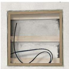
**4** Then use four frame dowels at the minimum to anchor the frame in the surrounding masonry. The next steps then follow the „Installation in drywalls“ instructions.
