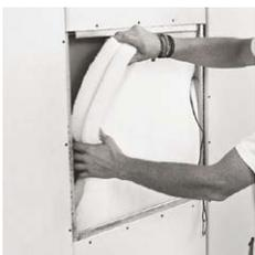
**5** Insert the cavity insulation material into the recess. For this purpose use the material enclosed.
