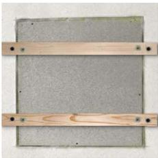
**3** With the help of two roof battens the frame can easily be brought into position and then fixed. Use construction foam to foam out the lateral joints and wait until the frame sits firmly and stable in the recess.
