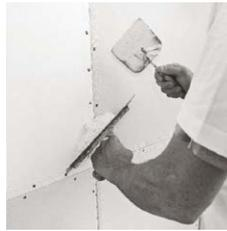
**7** The sealing and spackling of joints and edges as well as screw heads is effected using a flexible fine filler as it is usually applied in drywall constructions.
