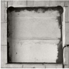
**1** For the installation of the invisible cerasonar speakers an mounting frame is required. This special accessory is available for all models. For this purpose an appropriate recess has to be prepared in the masonry. The recess has to be about 2mm larger all-round. Place the mounting frame into the recess to control the correct fitting.
