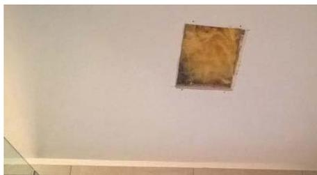
With help of the enclosed template the cutout is specified and then worked out by means of a rasp with cutter edge or a knife. Caution! Make sure that no power cables run behind the opening! The wiring to the speakers is to be effected via the existing openings, as e.g. of the built-in lights of ceilings or walls. Possibly additional holes are required which have to be closed again after cable installation.
