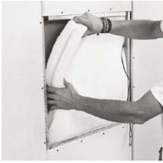
**1** Before the installation is carried out in walls or ceilings, the construction should be tested for vibration noise. Light beats with the heel of your hand against the plasterboard shell reveals any weaknesses of the substructure. The cavity behind the panel must get an insulation, for example, mineral wool or according to the specifications of the architect.
