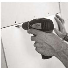
**4** Screw on the speaker according to the pre-drilled holes. The heads of the drywall screws should immerse about 1 mm into the diaphragm material. Since the diaphragm has a lower density than the plasterboard panels, it's essential to tighten the screws very cautiously.
