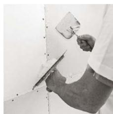
**11** Joints and screw holes have to be sealed using a fine filler.
